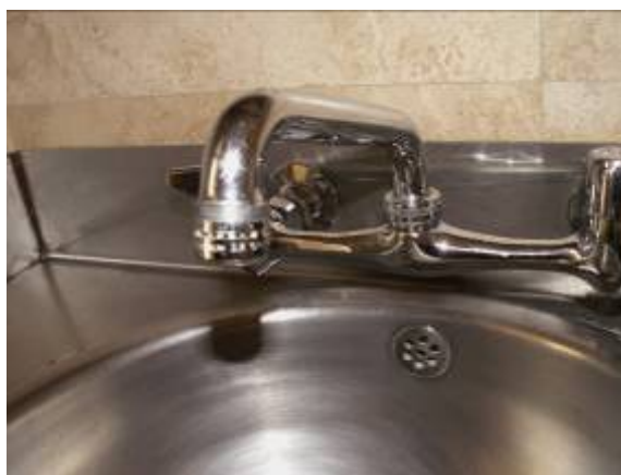
Figure 7. Many faucets at the Raleigh did have 2.2 gpm aerators installed as shown (right and left).
