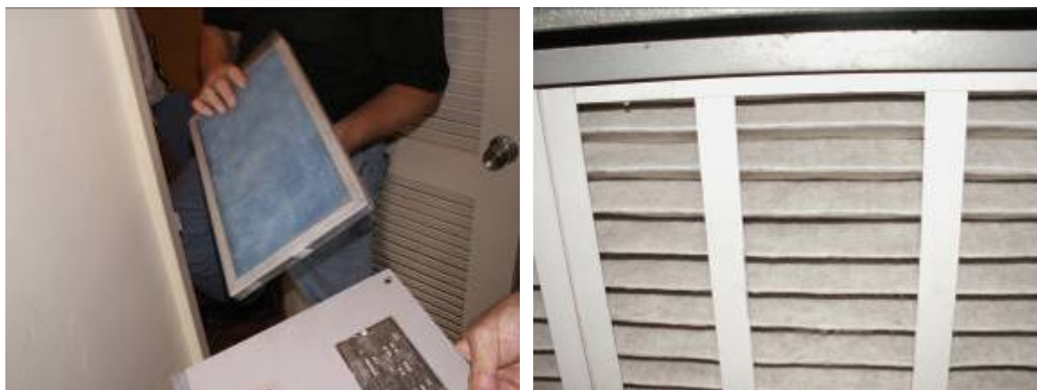
Figure 77. MERV 6 blue filter media cut to fit for the Raleigh individual HVAC units in the guest rooms (left). The Standard also uses MERV6 pleated media filters (right).
