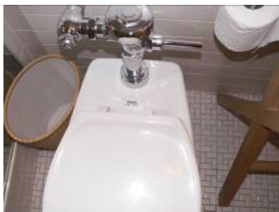
Figure 6. Typical flushometer style toilet in the Standard.
