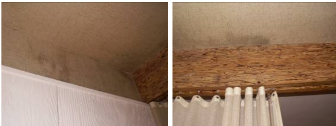
Figure 85. Visible mold/mildew staining in the Standard guestrooms.
