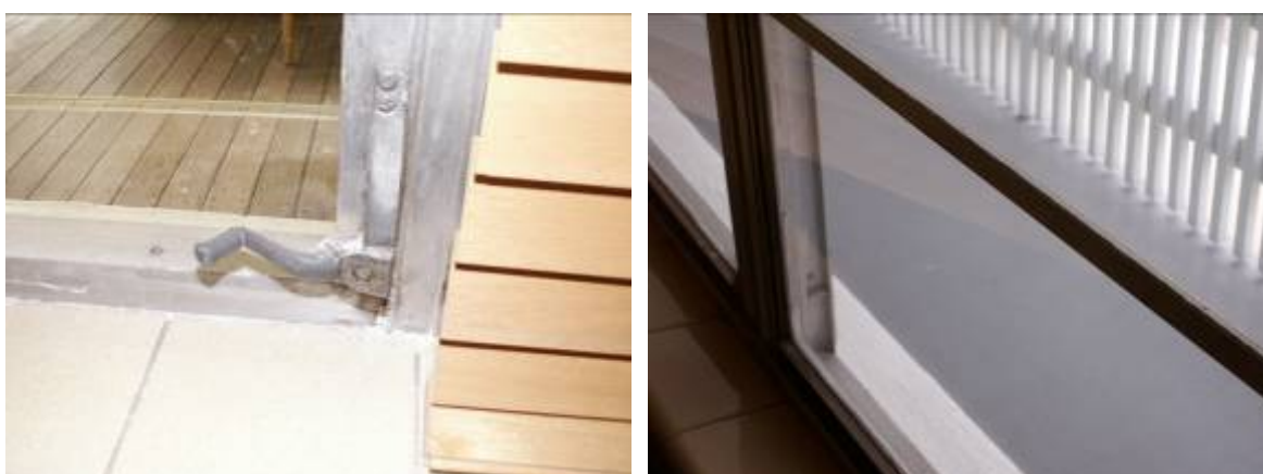
Figure 44. The Standard operable windows with hand crank on east side of the property (Left). The west wing of the Standard Hotel has different window style (Right).
