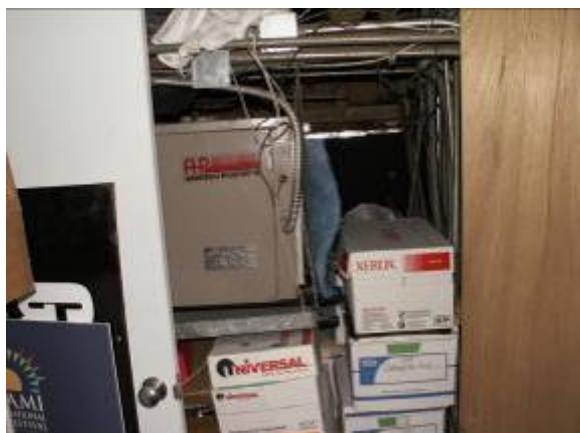
Figure 82. Mny of the air handler closets in the Raleigh are used as storage areas and are obstructing the flow of air to the units.
