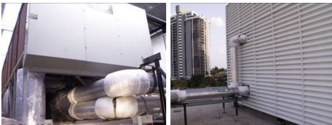
Figure 18. Air-cooled chiller heat-exchanger roof mounted HVAC unit at the Standard.
