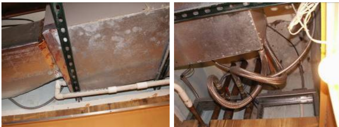
Figure 17. Typical heat pump unit in one of the Raleigh guestrooms.
