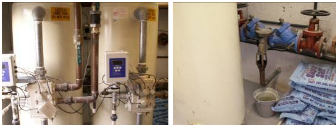
Figure 24. Water softening system at the Standard (left), and leaky line from the wall (right).
