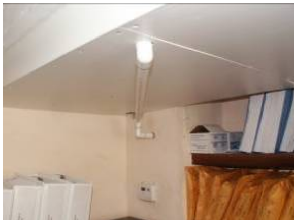
Figure 80. Exposed condensate drain running just above a work station in the accounting office. Note programmable thermostat controller for the space.
