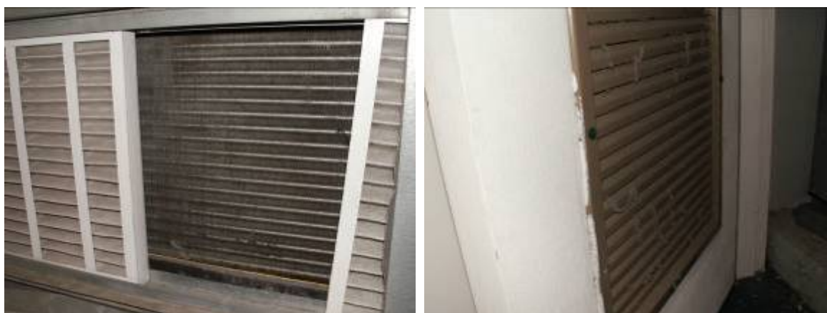
Figure 83. Air handler coils exposed prior to a mold test performed by the research team. This unit is located in the staff office of the spa area in the Standard Hotel. Note the caked on dirt on the inside of the vent grill (right).
