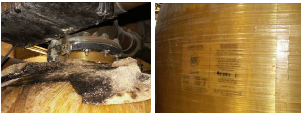
Figure 22. Non-functional water treatment system for whole building. The unit is leaking (left) and the fiberglass backwash tank (right) is thought to contain filtration media but the tank is not serviceable.
