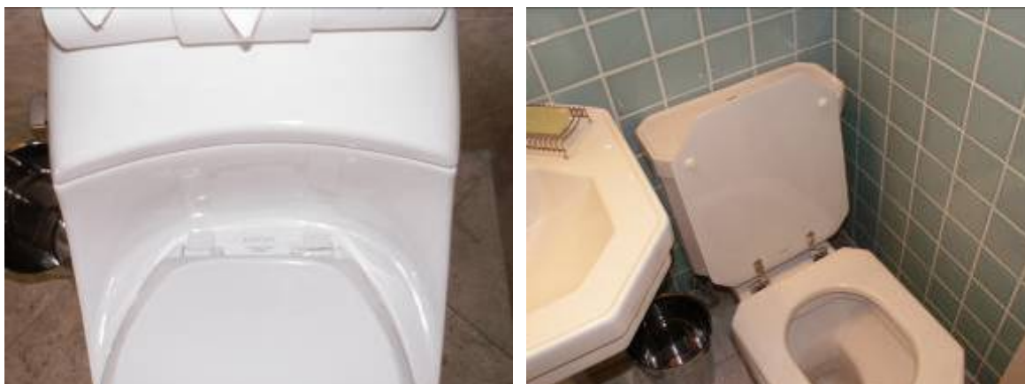
Figure 5. Typical gravity bowl one-piece toilet in the Raleigh (left). Typical gravity bowl two-piece toilet in the Raleigh (right).
