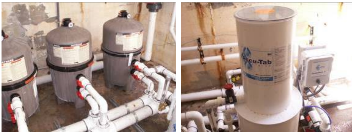
Figure 20. New pool filtration and disinfection equipment for the outdoor pool and water features at the Raleigh.
