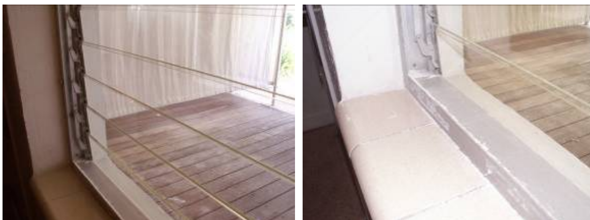
Figure 43. The Standard jalousie windows with visible condensation.
