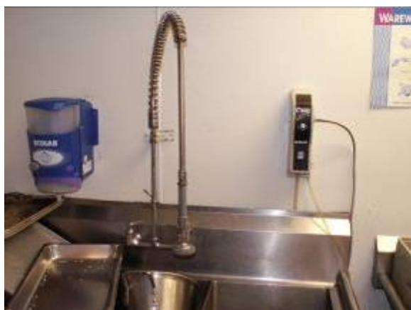
Figure 9. Spray rinse nozzle in the main Standard kitchen area.
