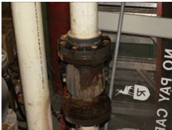
Figure 23. The lift station in the boiler room collects raw wastewater from the lower level to pump to the street manhole. The lines are visibly leaking as seen above.
