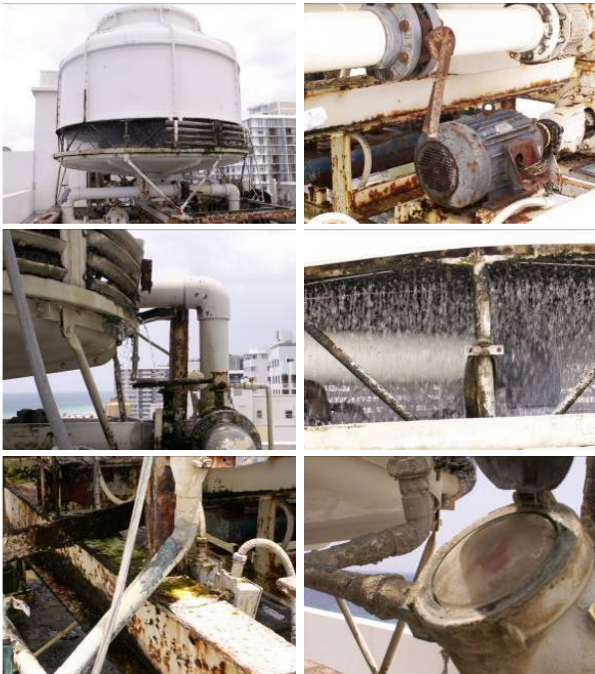
Figure 15. State of disrepair of the Raleigh roof chiller unit (June 2008). Top left: existing unit. Top right: extreme corrosion has taken its toll on the drive motors. Middle left and right: evidence of extreme amounts of water leakage over the sides and through the bottom of the pan. Lower left: algal growth, extreme corrosion,
