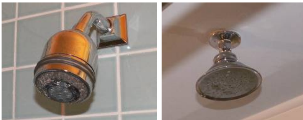
Figure 10. Typical showerhead in the guest rooms at the Raleigh (left). Note that the high hardness in the water has led to visible scaling. Typical downpour style overhead shower fixture at the Standard (right).
