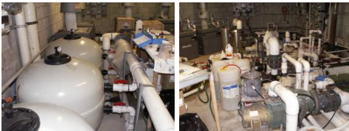
Figure 21 New pool filtration and disinfection equipment saline infinity pool at the Standard.
