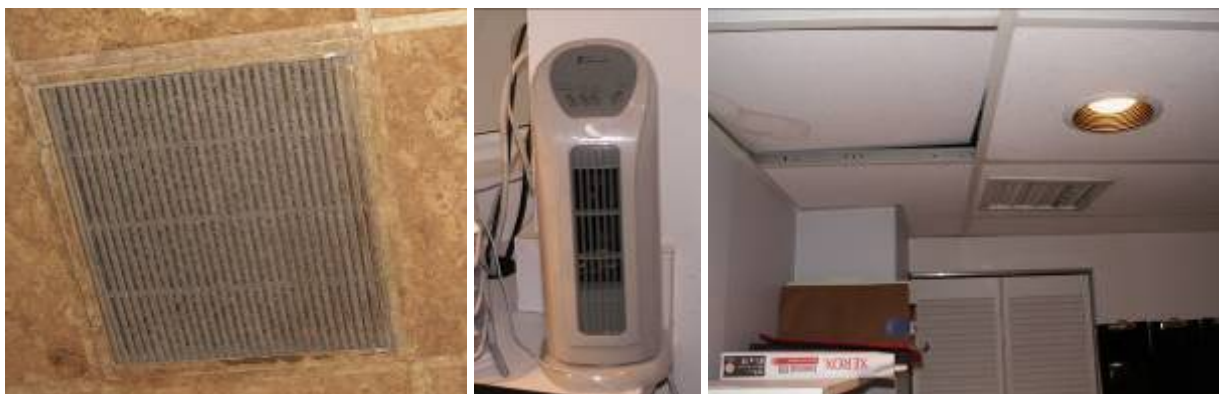
Figure 81. Note the amount of dirt coating the air vent grill (left). Air quality in the office spaces at the Raleigh has some workers bringing in their own air purification systems for their desk areas (middle). Evidence of water damage and mold/mildew stains and growth on the air ven grill (right) was spotted during the survey.
