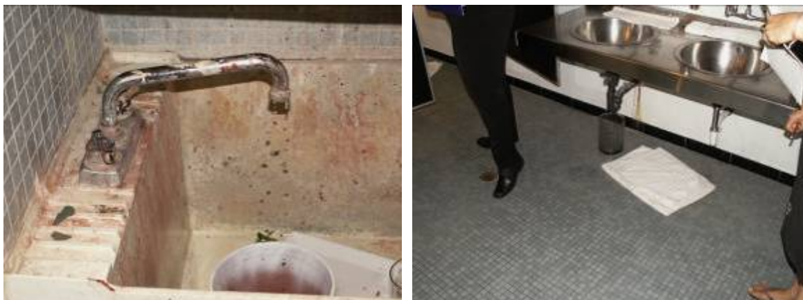
Figure 8. Leaking faucet fixture in one of the janitorial closets at the Raleigh (left and right).
