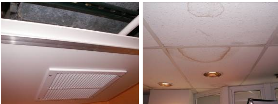
Figure 79. To deal with water leakage (right) and noise/rattling issues, plastic panels have been cut and placed under the drip pan in guest room units at the Raleigh (left). This has the effect of blocking the air flow in the closet into the vent, forcing warmer plenum space air into the air handler unit.
